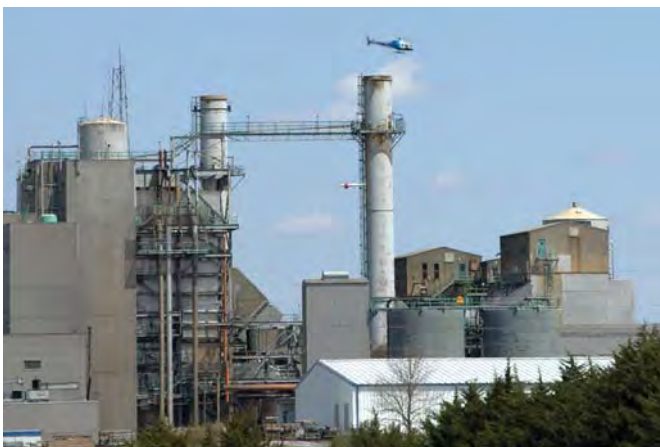
The HEM survey is conducted around the Sheldon power plant near Hallam, Nebraska.
