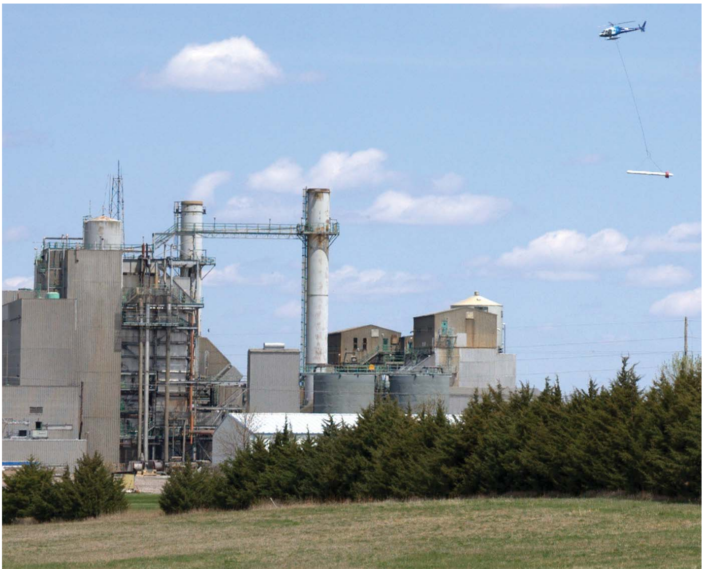
HEM survey being conducted near the Sheldon power plant north of Hallam, Nebraska.
